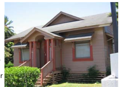
Telephone Exchange Building
